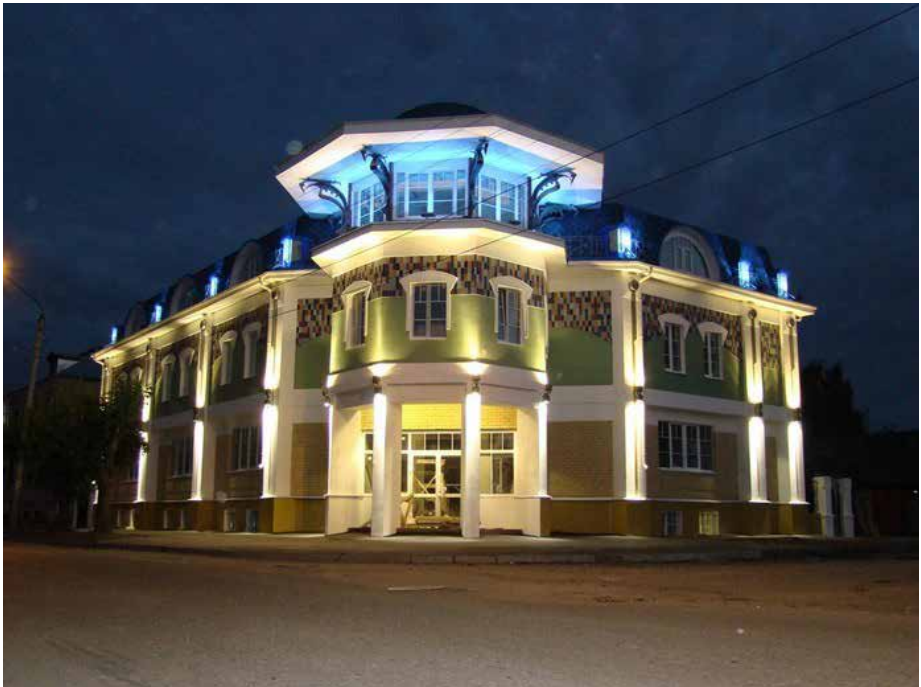
Pic. 2. Local lighting of the building [5].
